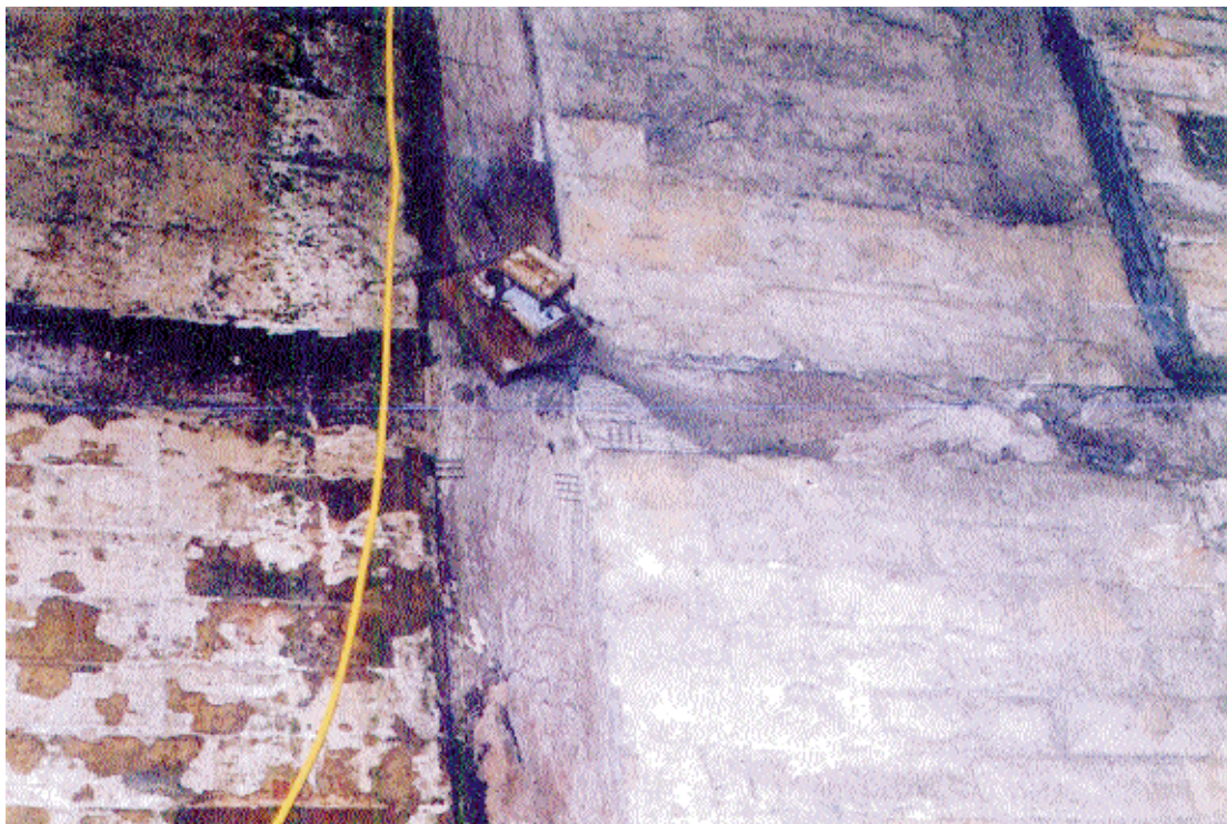
Plate 4. Building 1 Carpenters marks III and IIII, External west wall, Looking E.
