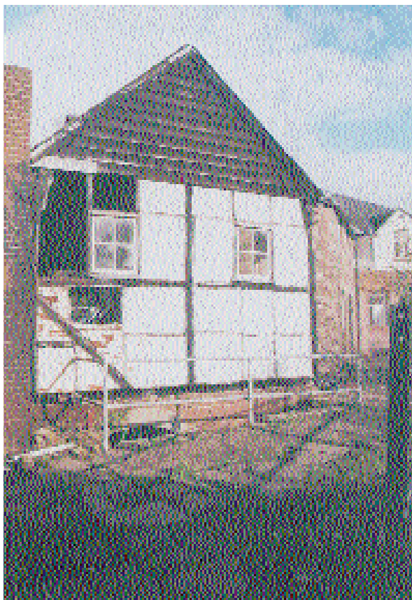
Plate 1. Building 1, southern elevation, Looking NE.
