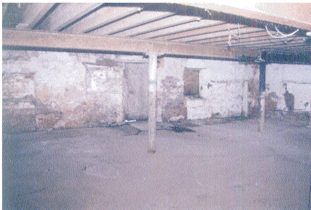
Plate 6. Building 2 Basement, eastern elevation, showing blocked doorway and window.
