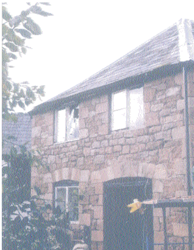
Plate 21. Building 6, eastern elevation.
