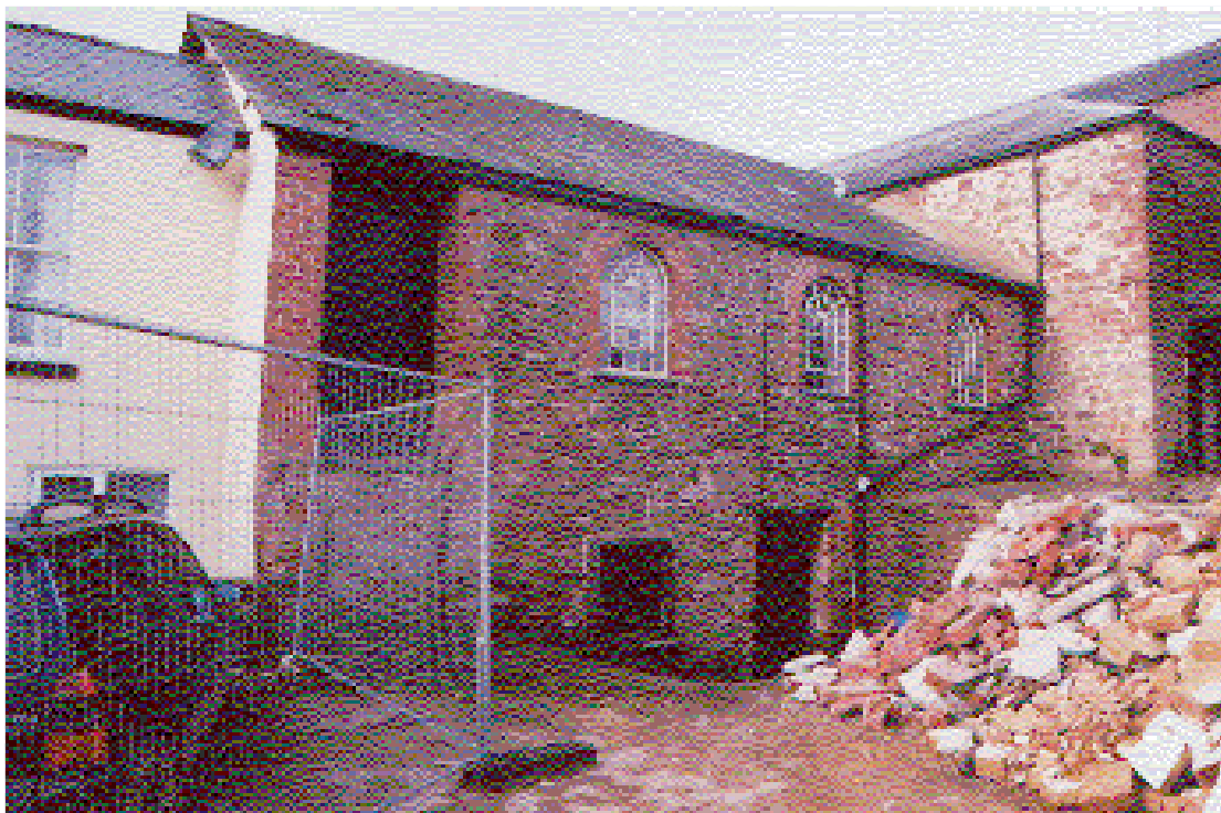
Plate 5. Building 2, Looking NW, Scales: 2m.
