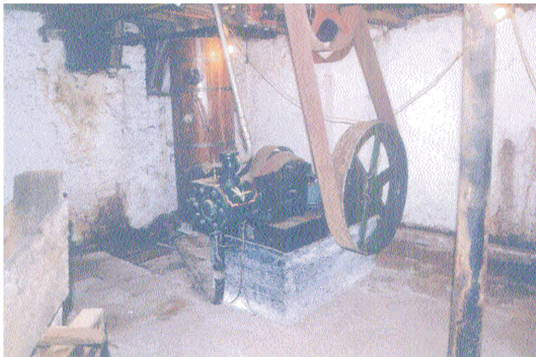
Plate 16. Tangye Steam engine and boiler, Building 4, Basement, Looking NE.
