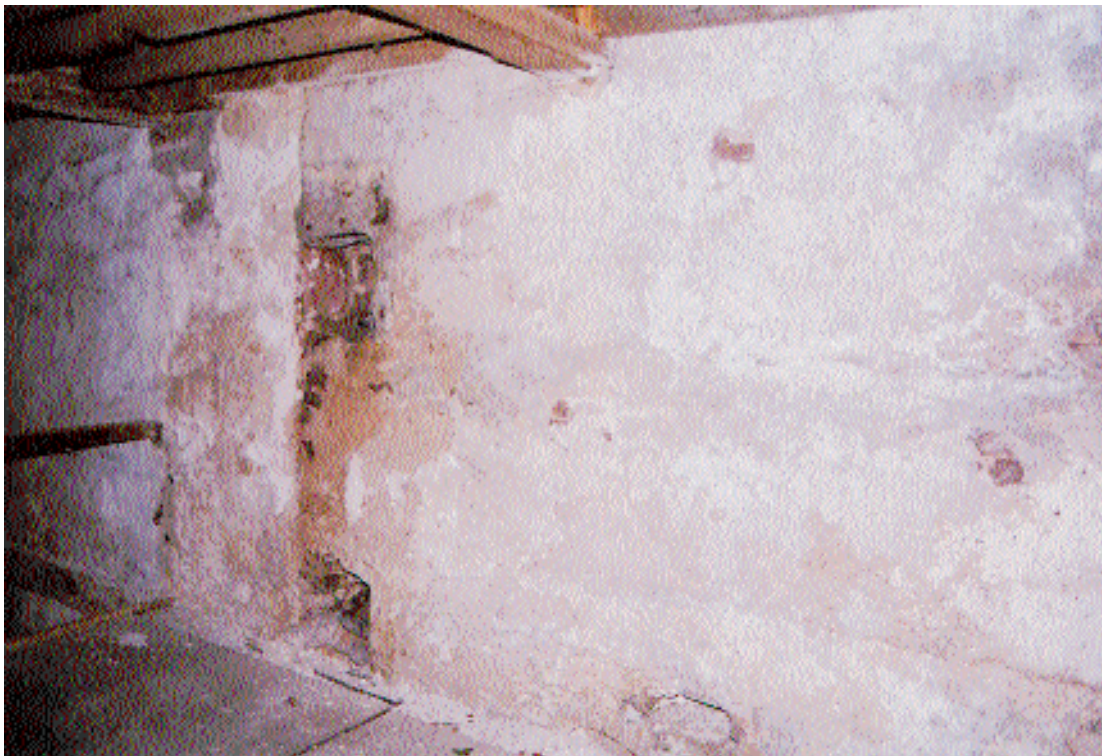
Plate 23. Quoin stones of Building 3 observed in south wall of Building 4, Building 4, Ground floor, Looking SE
