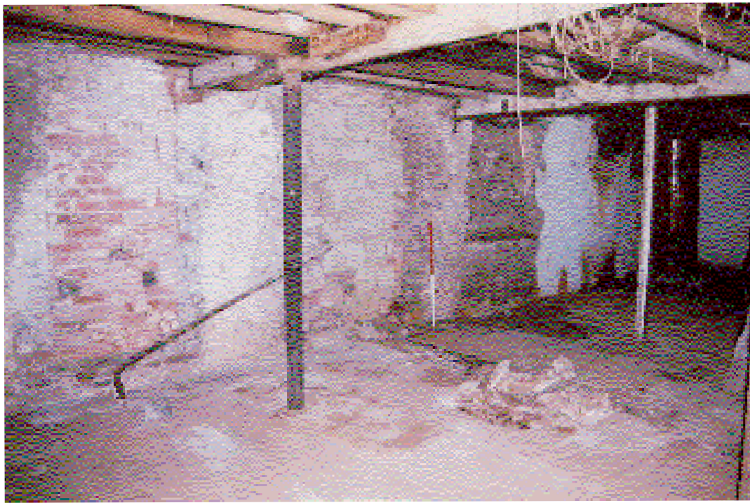
Plate 15. North Wall, Building 4, Basement, Looking NE, Scales: 1m.
