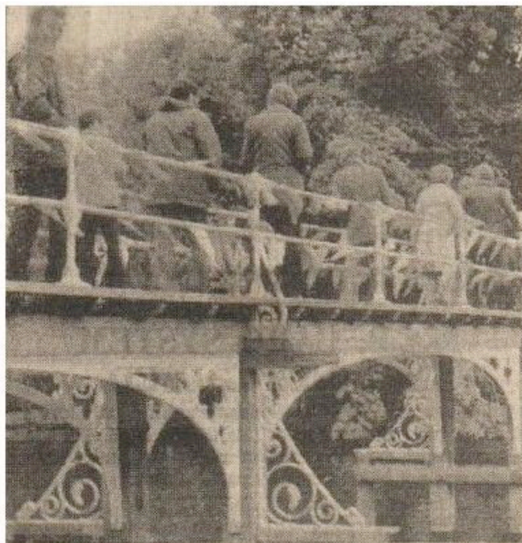
Part of the footbridge showing some of the elegant copy castings made at Herbert & Young's Foundry in Cinderford.
