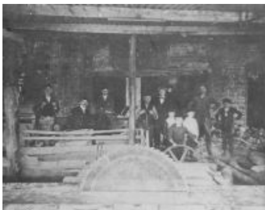
View of the Sawmills at Hale and Co. in about 1918, wooden boxes were nailed up by boys for packing tinplate, and a portable steam engine drove the saw. The plant was accommodated in buildings originally houses, then offices, and afterwards stables for the New Bridge Pits, the capped shafts of which are in Hale's yard
